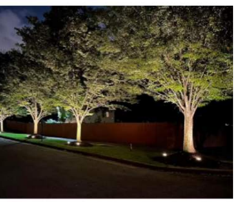
D TREE ACCENT LIGHT • IN-GRADE LOW OUTPUT FIXTURES WITH GLARE SHIELDS THROUGHOUT LANDSCAPING AREAS
